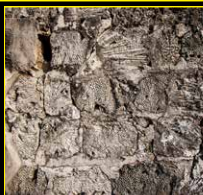
Jaffna Fort. Now in the process of restoration and repair. The rubble on the far left is from the destroyed old Dutch church. The coral 'bricks' (above) reveal the masonry used to build the fort - seen on walls and on some steps. The well which has been cleaned up has a history of being haunted with the reflection of a Dutch girl seen by some in the water. The stone archway steps have escaped the destruction of the war years - thankfully! It will be many years before full restoration is completed.
